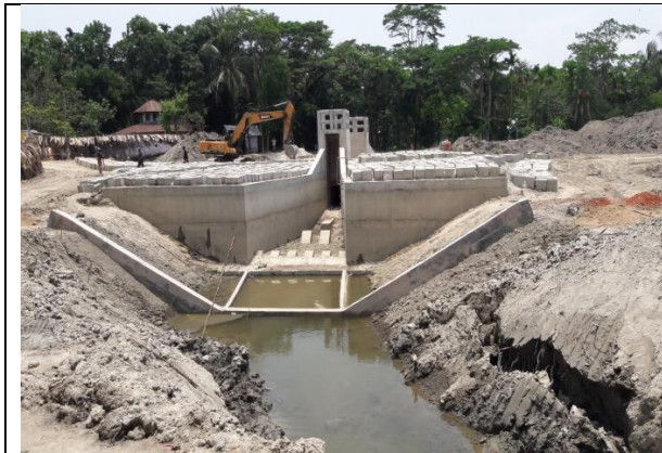
DS-2 under polder 40/2, Gahorpur village, Patharghata Union, Patharghata, Barguna
