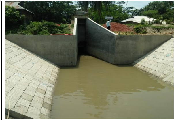
FS-1 under polder 41/1, Purbo Kawrabunia village, Aylapatakata Union, Barguna sadar
